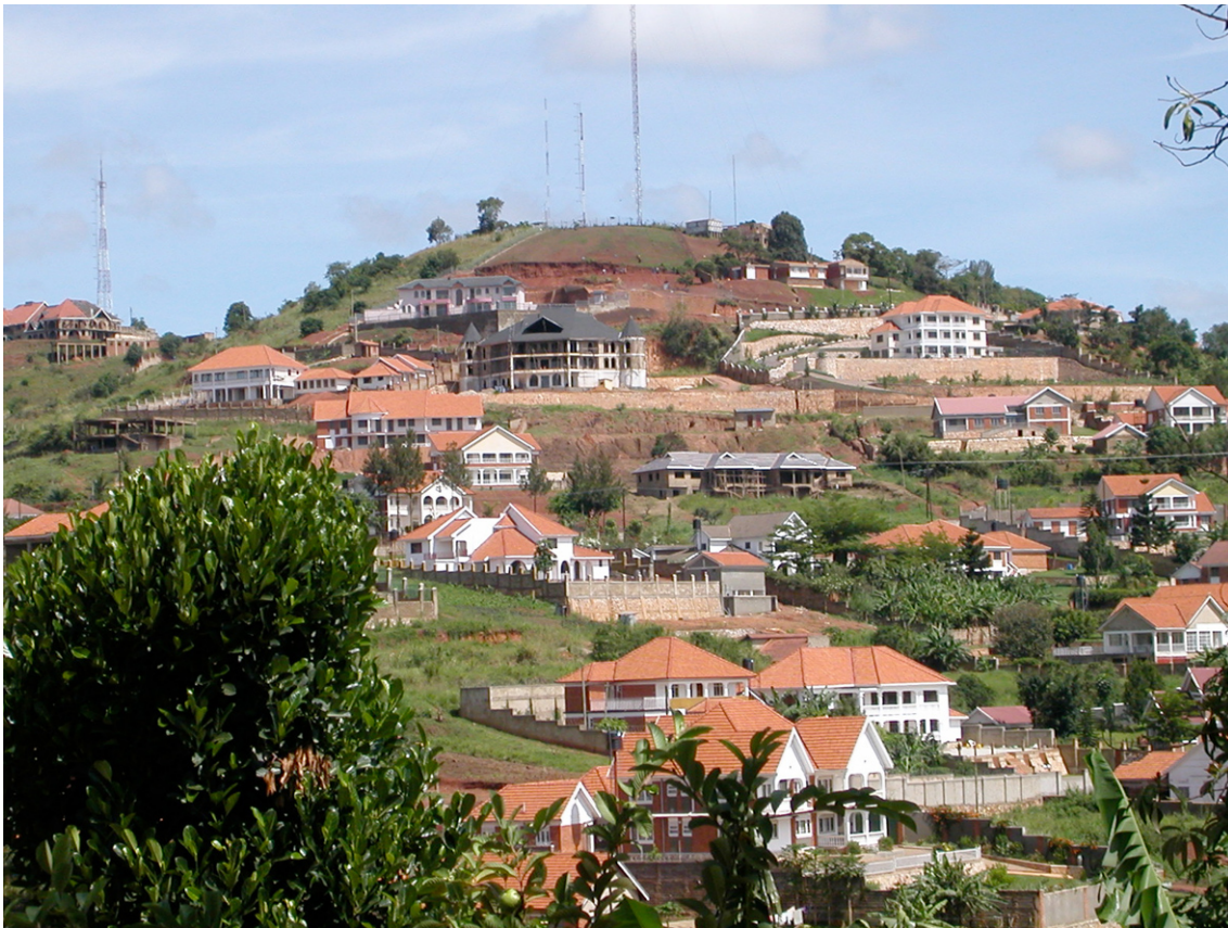
Figure 1: Housing on Naguru Hill, Kampala. Source: (Olweny, 2005)
