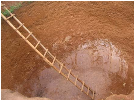
Figure 7: Completed Soakaway Pit. Source: (FBTA, 2006)
