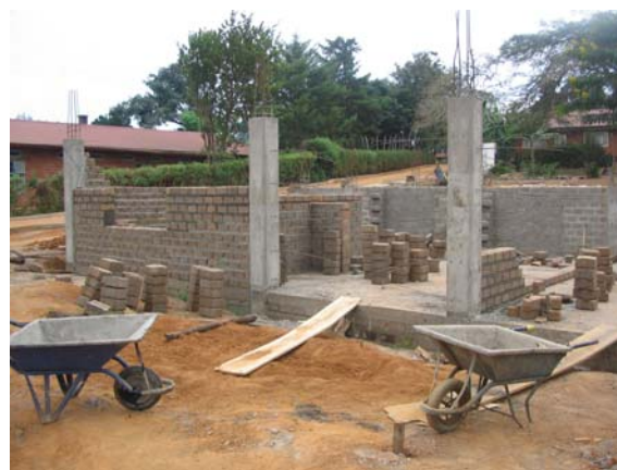
Figure 3: Classroom Block. Source: (FBTA, 2006)
