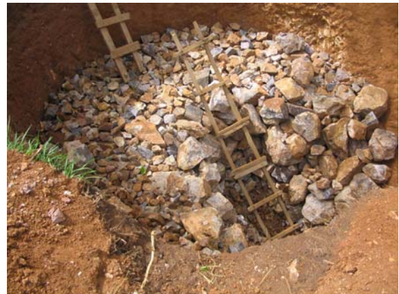
Figure 8: Soakaway Pit With Hardcore. Source: (FBTA, 2006)
