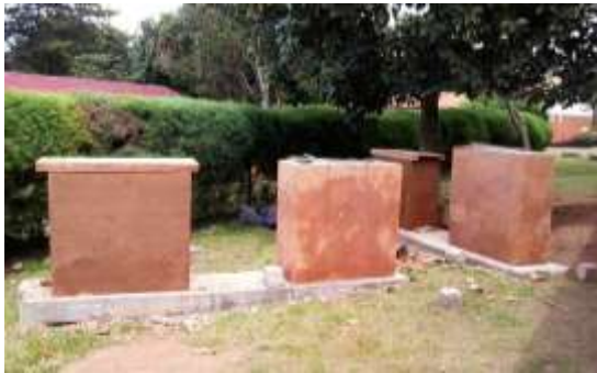
Fig. 3. The completed poured earth walls
