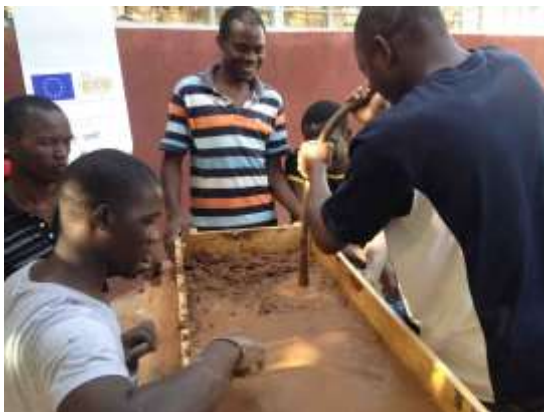
Fig. 2. Completing the first poured earth wall
